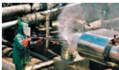
▲ High-pressure water jetting.
